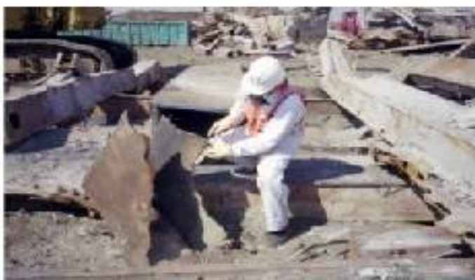
Fig. 1. A. Astaneh inspecting an internal column of WTC which has been hit with a round object
